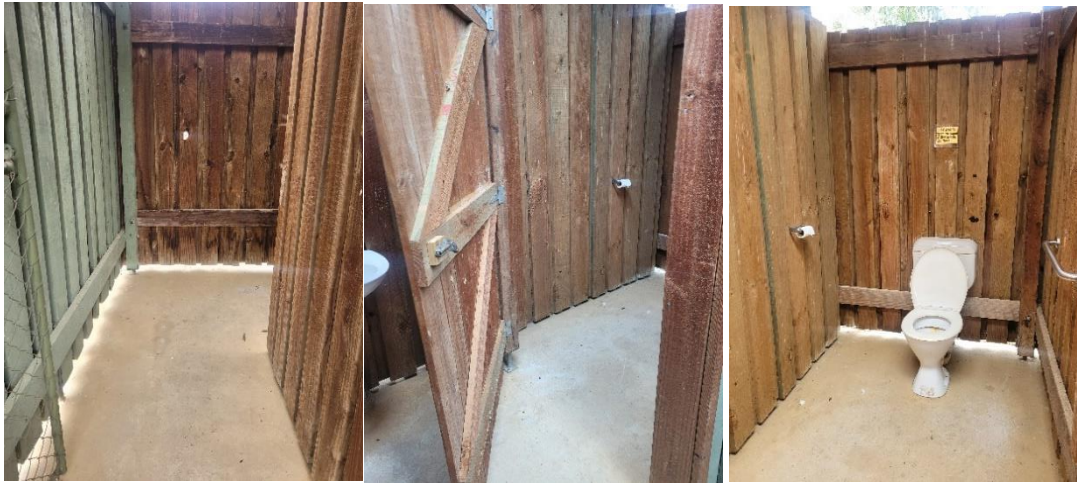
Caption: Entrance at 820mm, toilet cubicle entry at 560mm and women's toilet with handrail.
